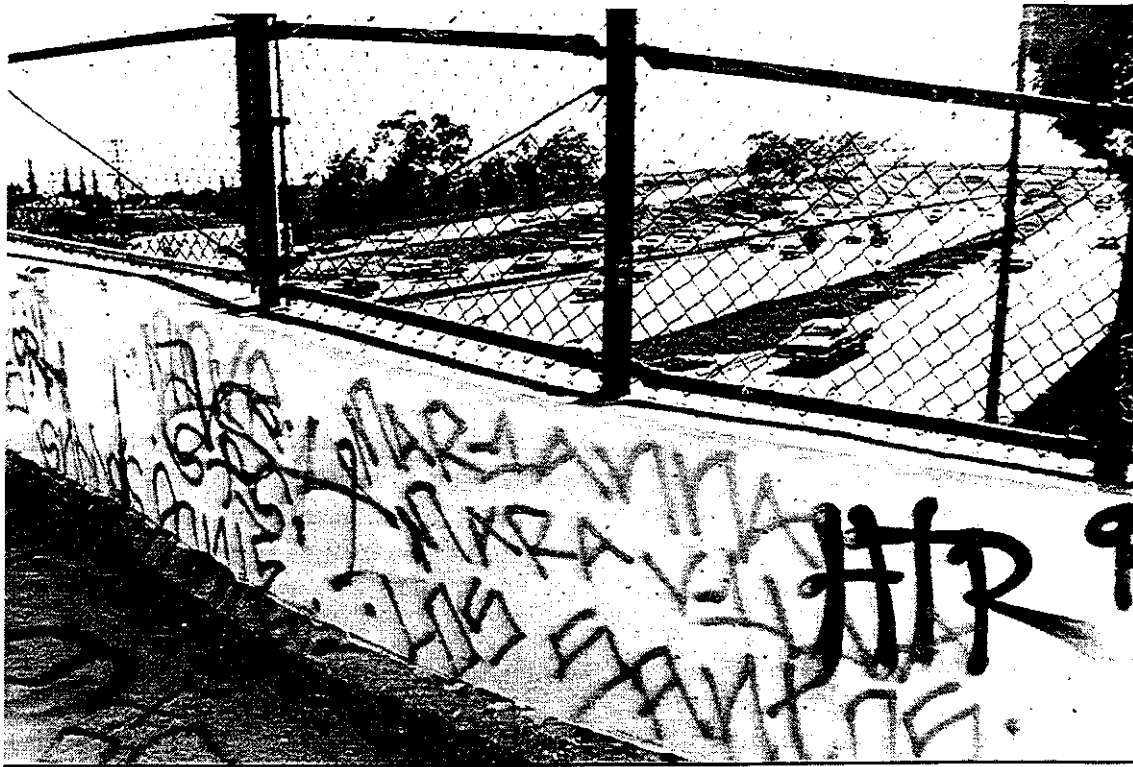
Freeway construction in the 1950's divided established communities on the East Side. Photograph: George Rodriguez
